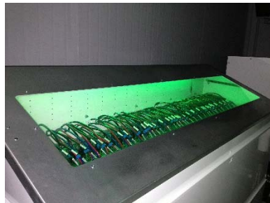
Servers and switches
